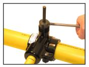
16 To allow flow through service, back punch up until the top of the punch is flush with top of saddle. It is important that the punch does not protrude above the top of the saddle tee.
