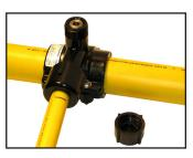
17 Verify that the O-ring is in the cap. Install cap on saddle hand tight. Do not use wrenches on cap.
