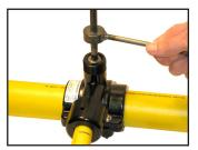
15 Screw punch down until stop on drive key contacts the top of the saddle tee. The tap is now complete.
